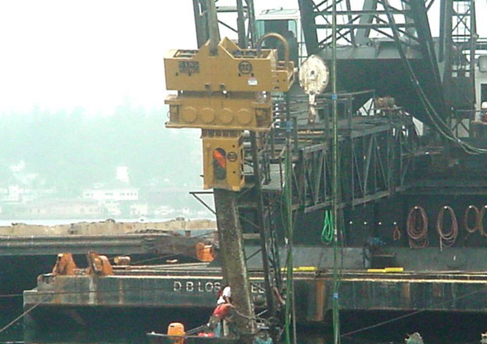
APE Model 400 in leads extracting Concrete Piles
